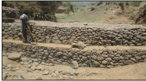
Figure 2: Check dam constructed in Goshwuha area to harvest water and sediments Source: Photograph taken during field survey, 2014
